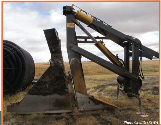
Tiling equipment and perforated pipe
